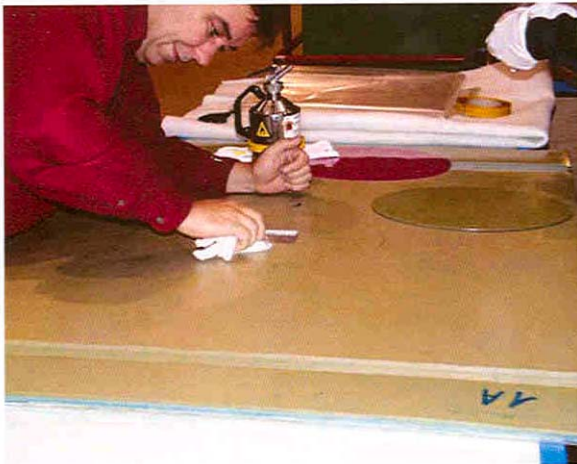
Cleaning of bonding surface
