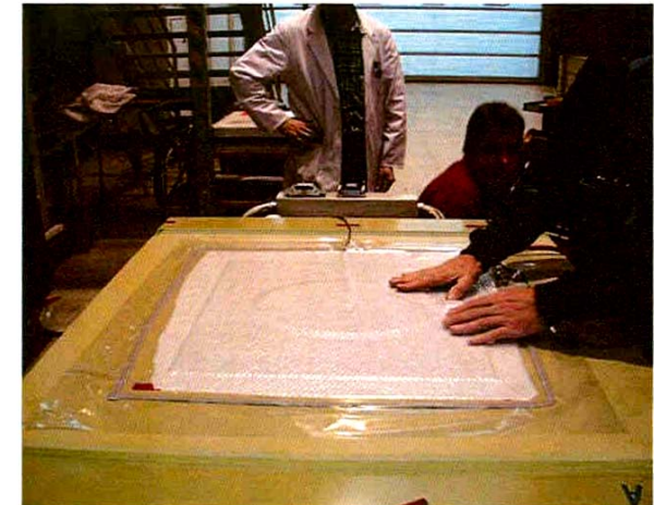
Application of vacuum foil, thereafter start of curing with Heatcom ® device, low vacuum pressure
